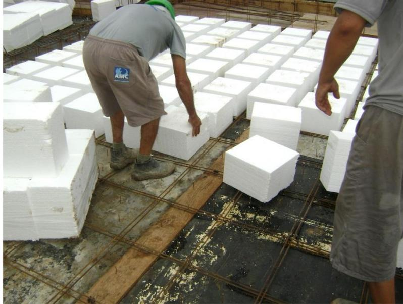
**Figura 1 – Laje nervurada com EPS [4]**
